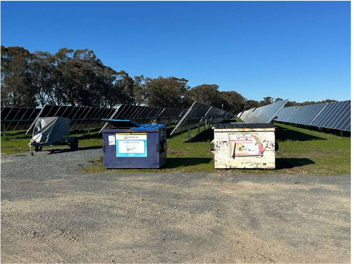
Photo 22 – Waste storage containers
