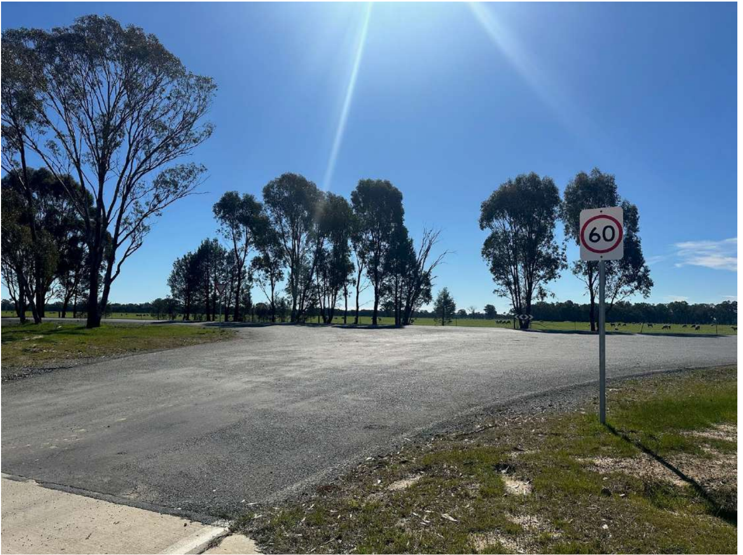
Photo 2: Upgraded intersection with Benambra Road
