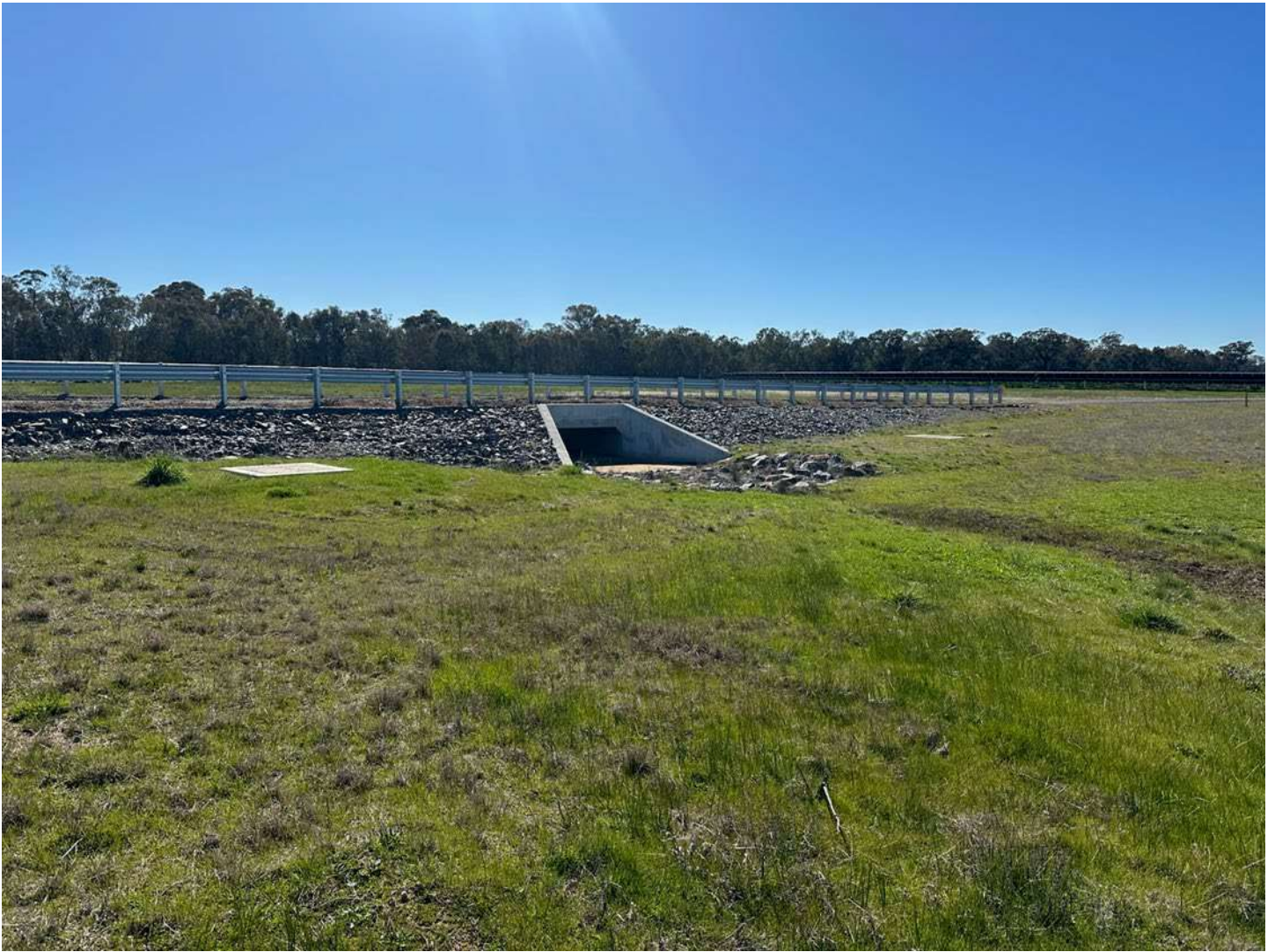
Photo 24 — permanent stormwater culvert and rock scour protection
